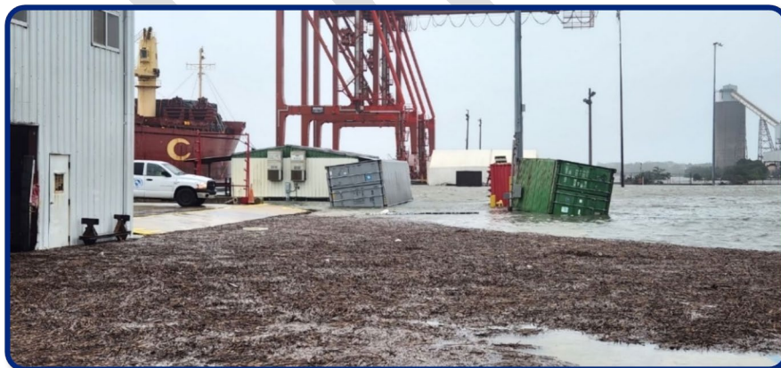
Source: Photo courtesy OHPA Staff, November 2022
