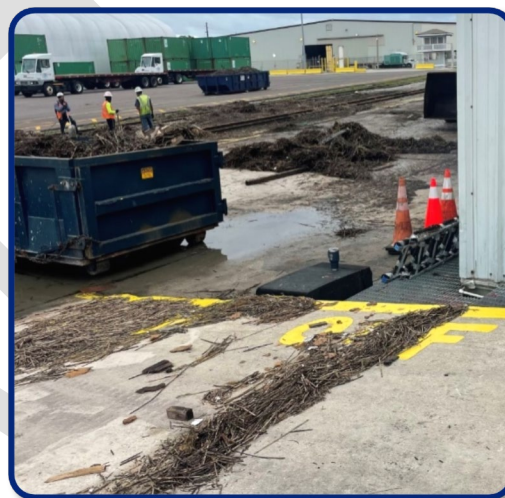
Source: Photo courtesy OHPA Staff, November 2022
